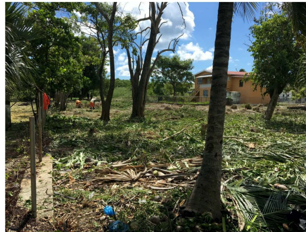
Cleaned Scout lot after a day of hard work by inmates of the Kolbe Foundation
