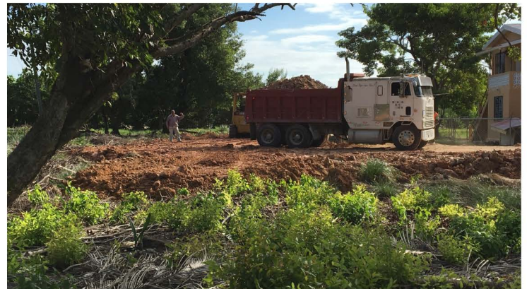
Dump trucks delivering clay fill to the Scout lot
